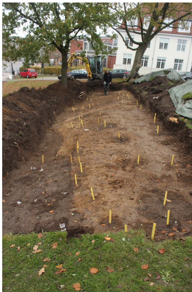
Figure 8: Parts of the excavation trench from 2017. To the North (to the left in the picture), the 1909 removal of the rampart that lay beneath it can be seen as a large, dark feature. Photo: Mads Runge.
